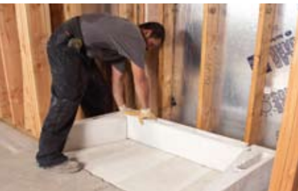
1. Installing base and first course
