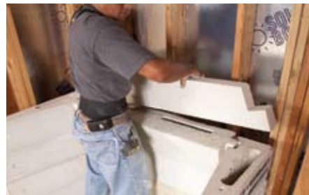
2. Starting the smoke chamber
